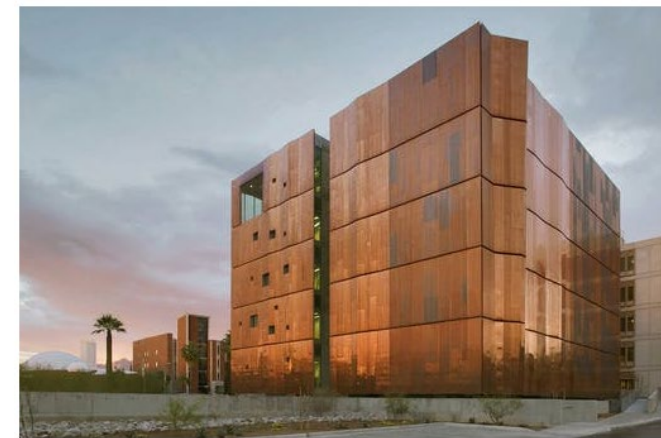
Metal cladding at the Meinel Optical Sciences Research Lab at the University of Arizona by Richard Kennedy Architects. The price of steel mill products has risen 108.6% in the last 12 months. Photo: Bill Timmerman.
