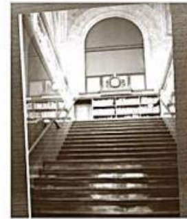
Original stairs and window
