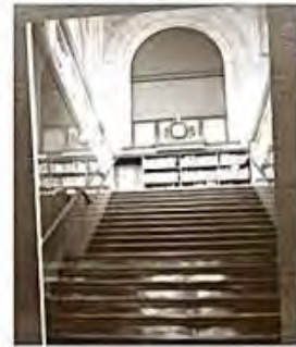
Original stairs and window
