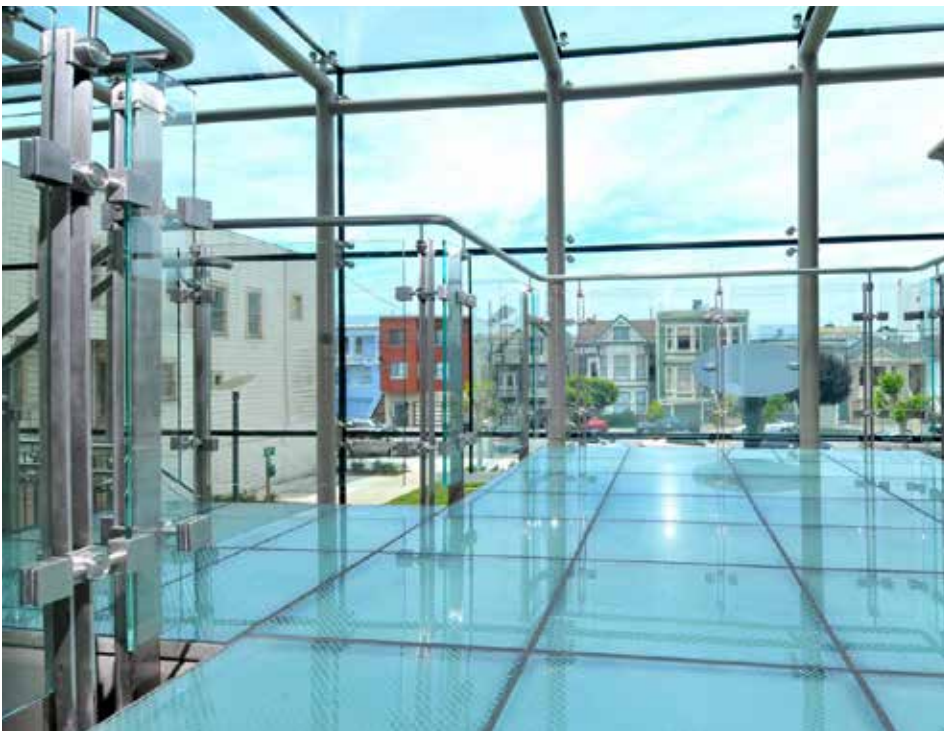
Upper floor of the addition to Richmond/Senator Milton Marks Branch post-BLIP
