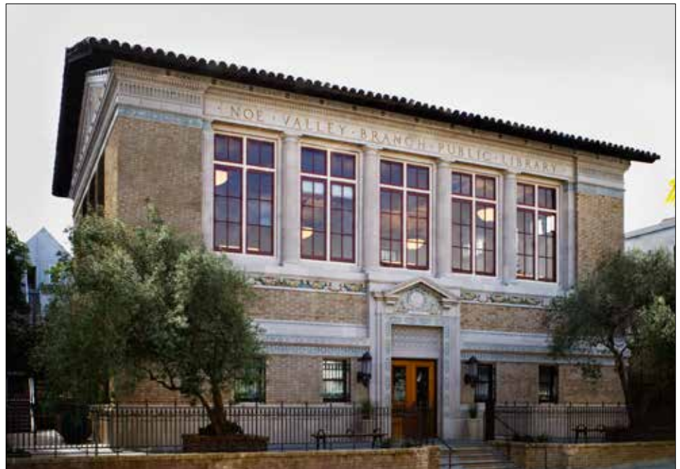
Noe Valley/Sally Brunn Branch post-BLIP
