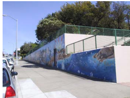
View of Retaining Wall to remain
