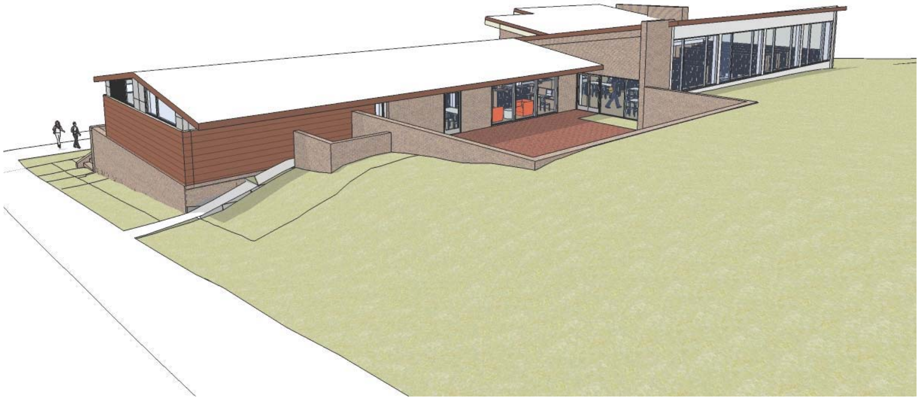
VIEW FROM NORTH
